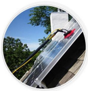
PV panel cleaning
